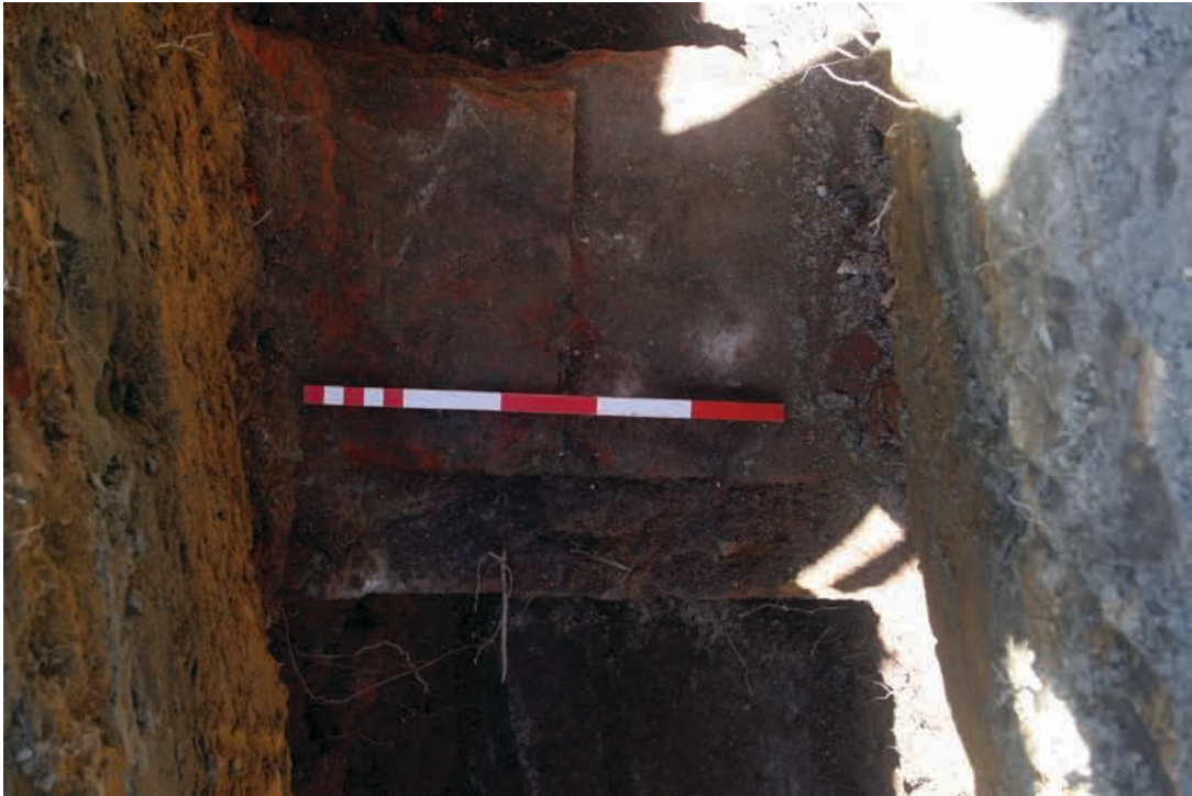
Figure 3. Brick footing/load bearing wall and later mesh-reinforced concrete facing, in the base of Test Pit 2.
